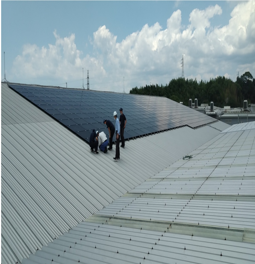
Installed solar panels on the roof of the 2 nd factory at Takaono in June 2020
