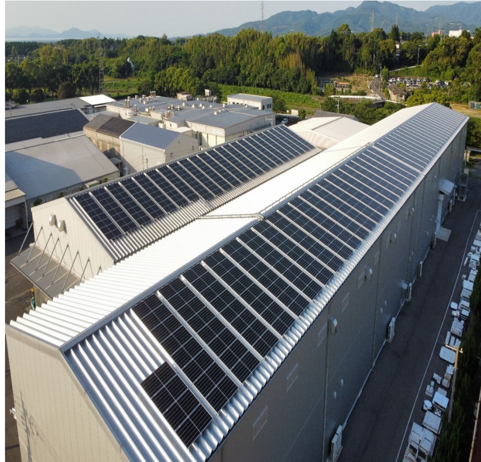
Installed solar panels on the roofs of the 4 th & 8 th factories at Takaono in June 2021
